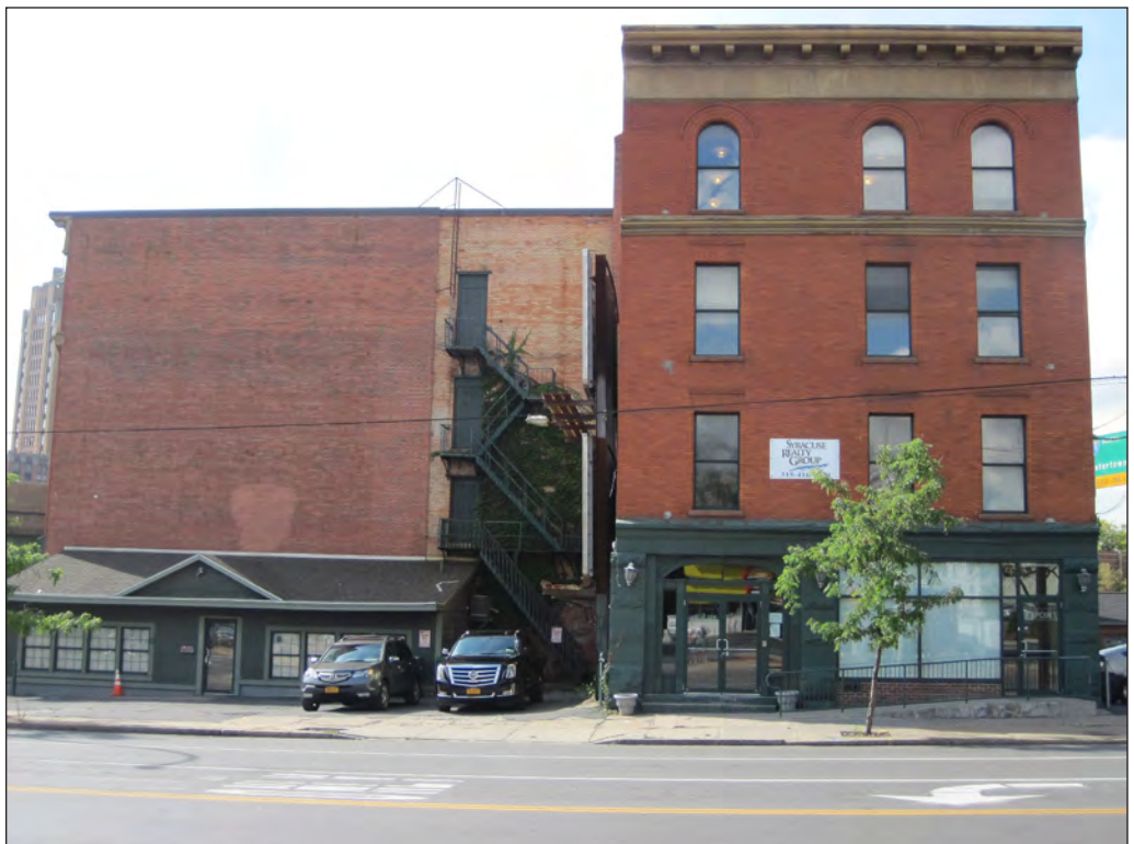
The east façade of the Crichton Apartments
