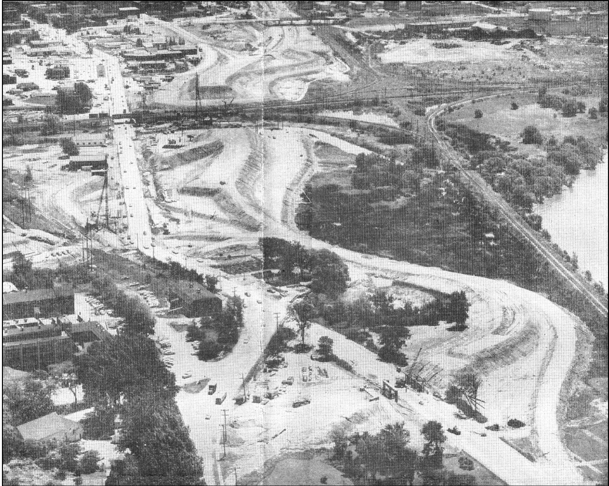
Figure 2.4.6-13. 1958 aerial photograph showing the construction of the northern portion of the Oswego Boulevard Expressway. Linking the Oswego Boulevard Expressway with Interstate 81 north of the city required significant earth disturbance and construction of earthen berms to navigate the landscape and poor soils closer to Onondaga Lake (Hoffman, 1958b; collections of the Onondaga Historical Association)
