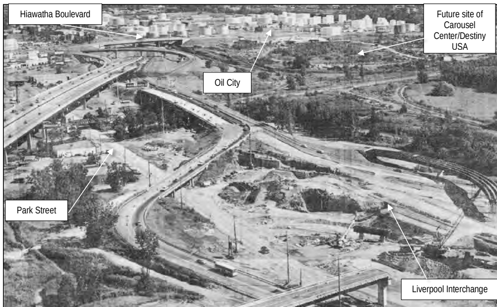
Figure 2.4.7-1 1985 photograph showing the reconstruction of Interstate 81 north of Hiawatha Boulevard at Liverpool Interchange. The reconstruction of Interstate 81 in the early 1980s involved significant ground disturbance associated with the realignment of the construction of a new viaduct over Park Street as well as a new Liverpool interchange. (SHJ, 1985; collections of the Onondaga Historical Association)
