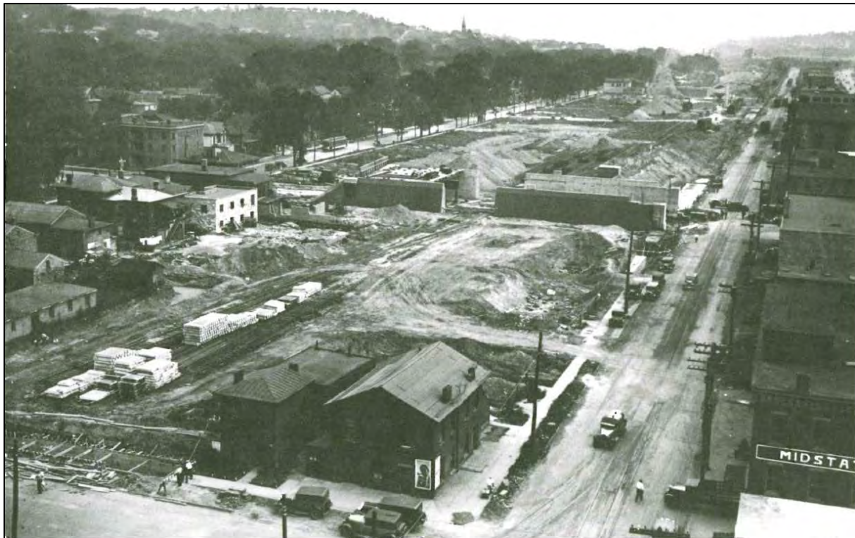
Figure 2.4.6-3. Circa 1935 view of construction of elevated railroad right-of-way. This circa mid-1930s view from McBride Avenue looking east depicts the construction of the elevated New York Central Railroad right-of-way between Burnet Avenue (depicted as a tree-lined street on the left of the frame) and Canal Street (on the right of the frame). Note the considerable ground disturbance as well as the houses that were later removed for construction of the railroad right-of-way, which was common within all parts of the elevated right-of-way that would later become Interstate 690 in the 1960s. (CNYCNRHS, 1986)
